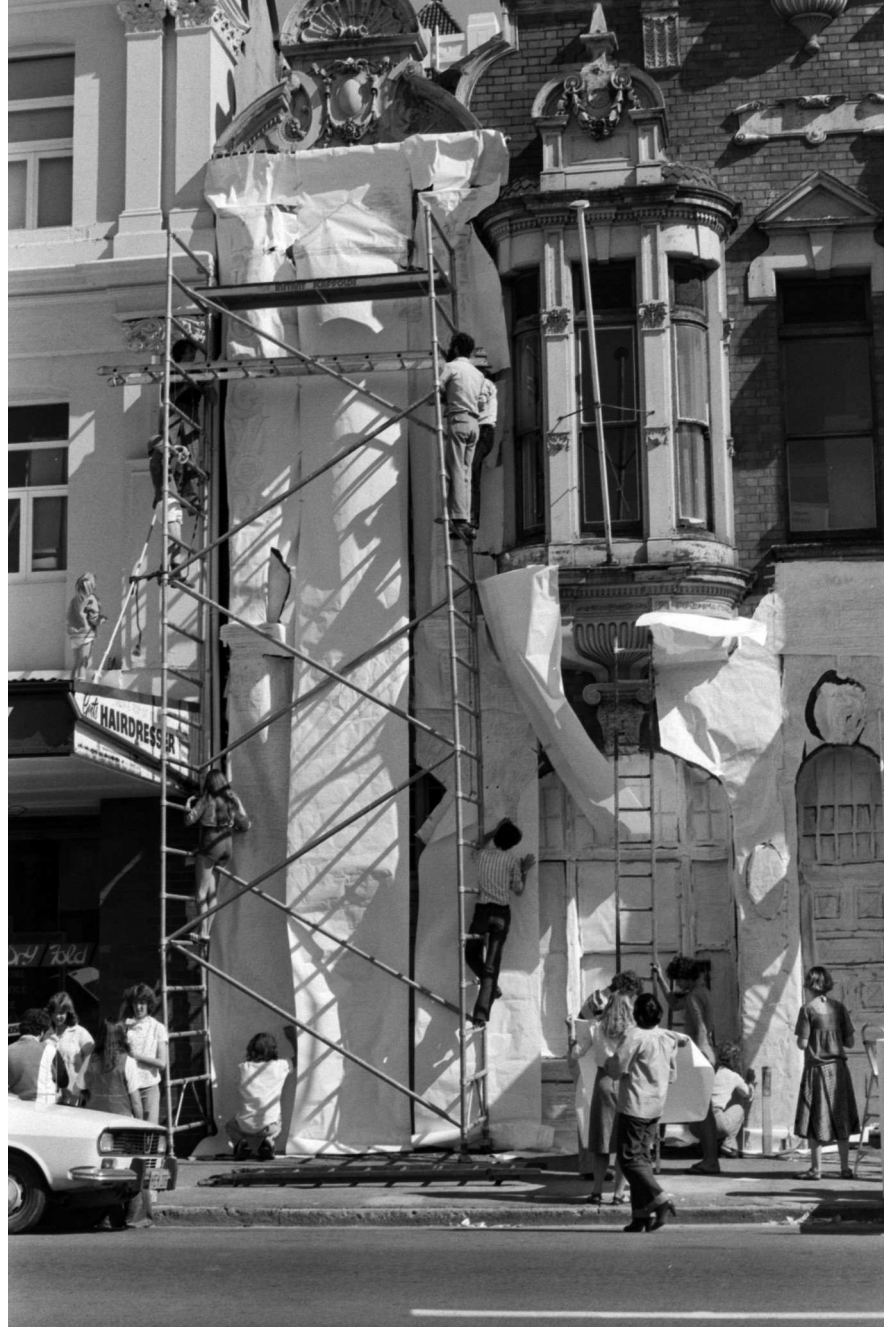
Simon still on the awning. Brian on the scaffold.
