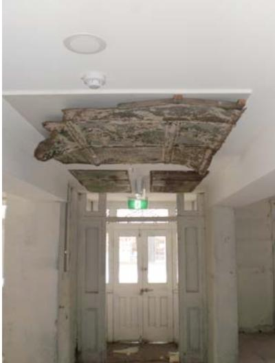
Figure 6. Sections of pressed metal ceiling and battens affixed to the new plasterboard ceiling.
